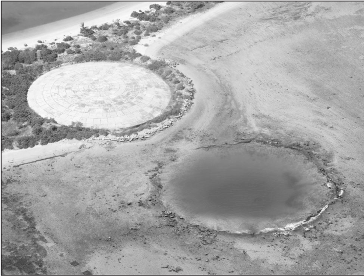
A TEST OF US INTEGRITY AND RESPONSIBILITY: The Runit Dome, a 350-foot wide concrete container built by the US to contain nuclear waste, leaks plutonium.
